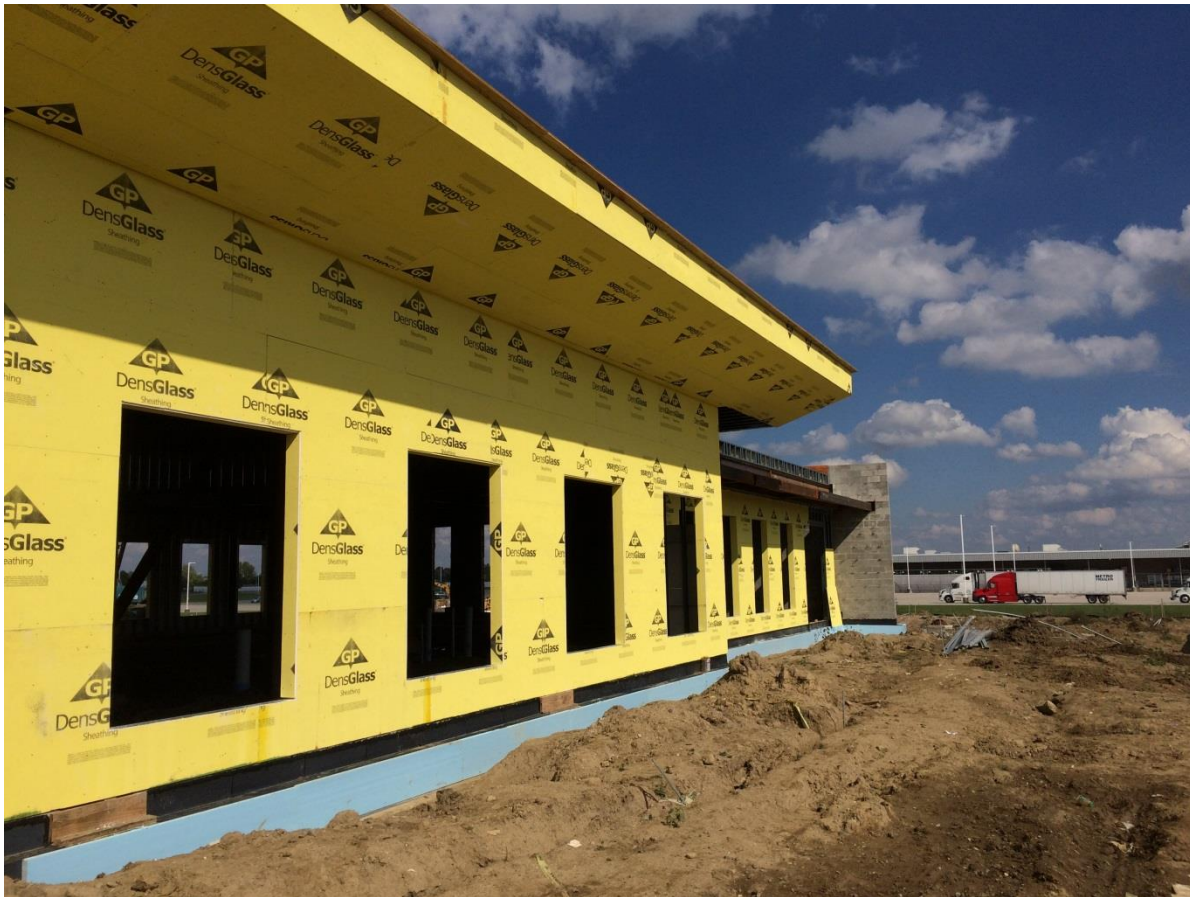
Project Site on October 3, 2018 View looking east of the south elevation and overhang.
