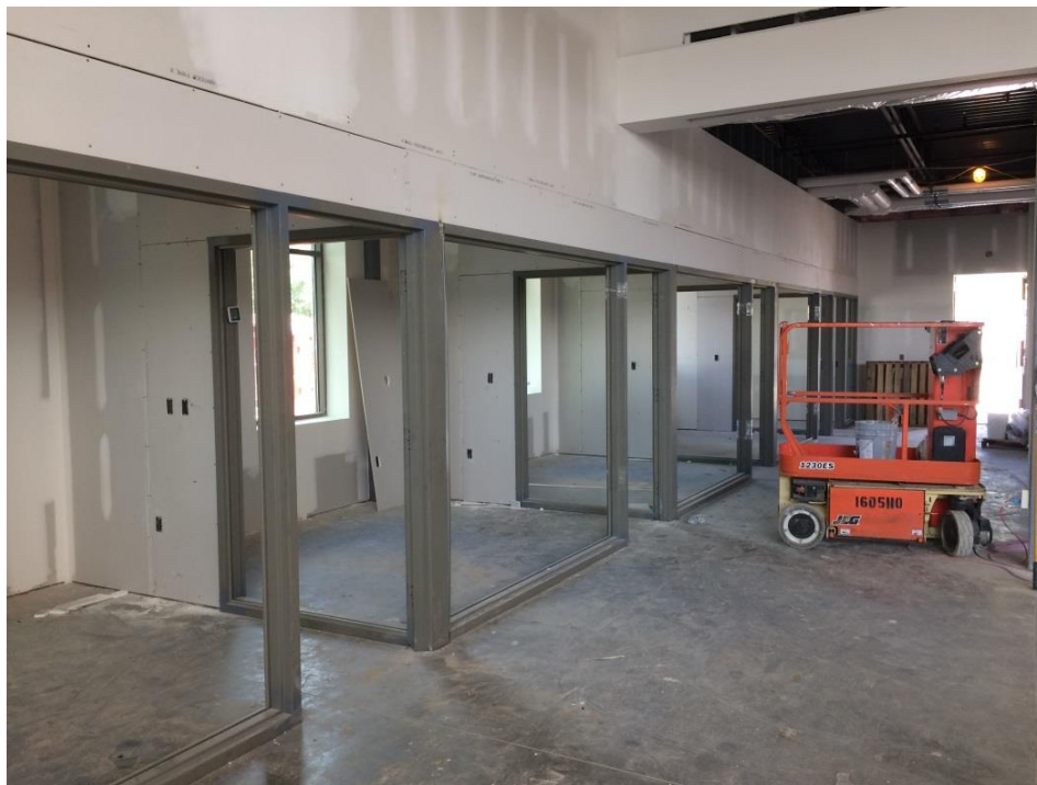
Project Site on October 3, 2018 New Study Rooms on the north side of the building.
